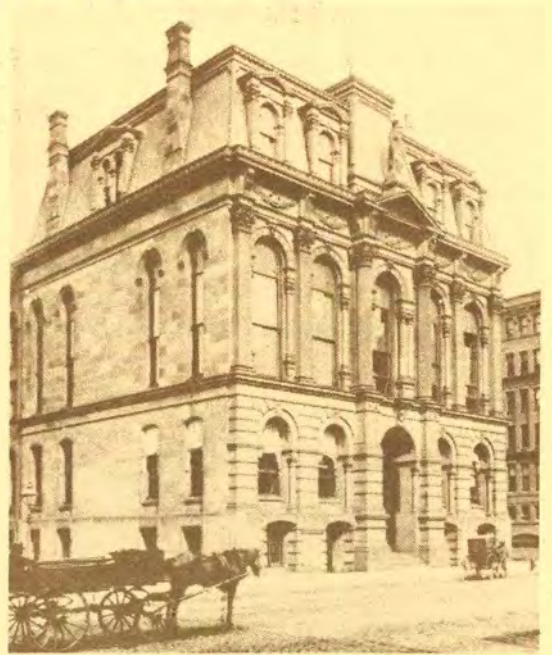
"OLD" COURTHOUSE ANNEX PHOTOGRAPH COURTESY OF THE CLEVELAND PUBLIC LIBRARY
